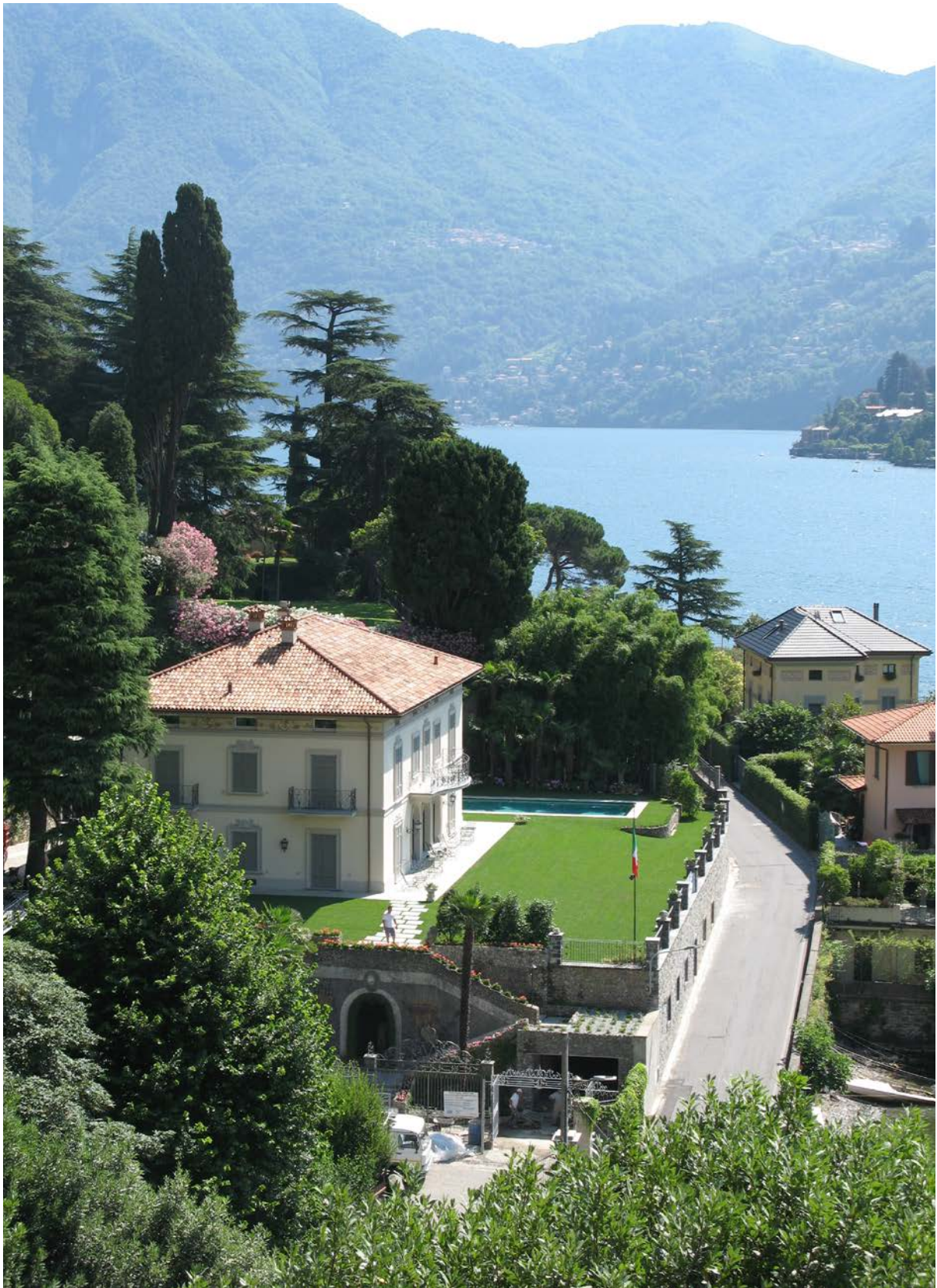
Private villa • Moltrasio (CO) Demolition, building reconstruction and new pool
