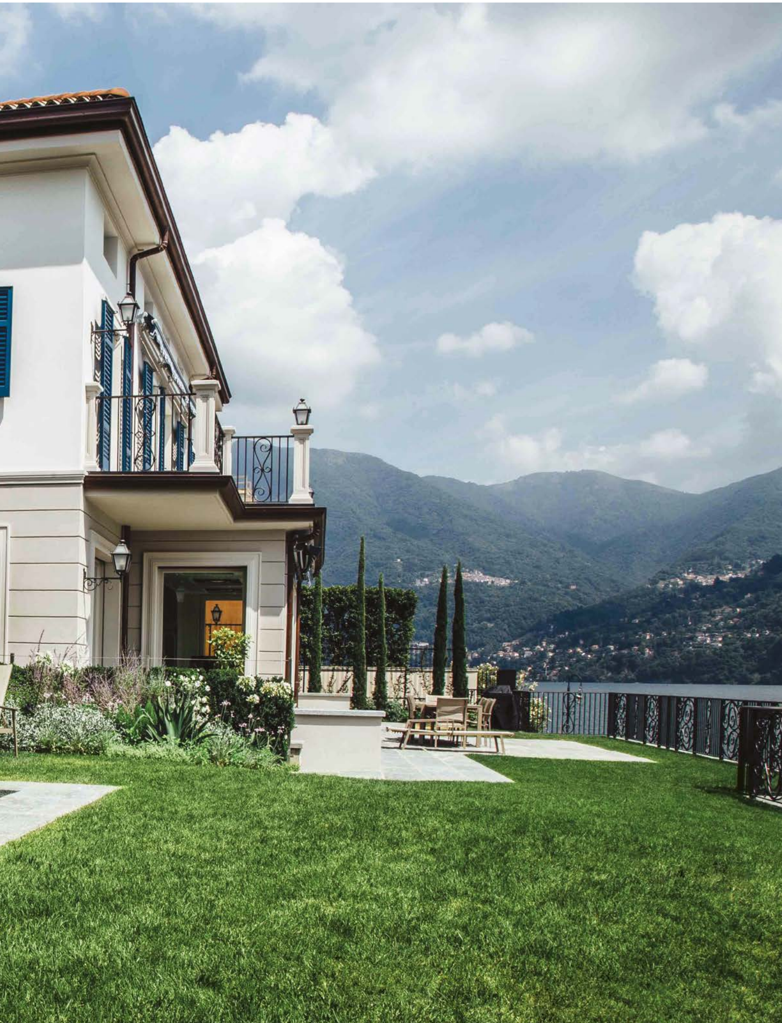
Private villa • Moltrasio (CO) Renovation of the villa, realization of internal boathouse, garden, pool and guardian' house, also renovated
